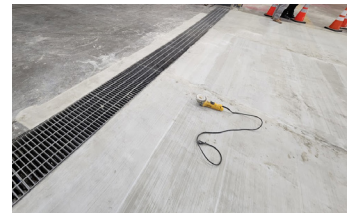
Finished repair ready for a coat of Ecobeton-USA Vetrofluid®.
