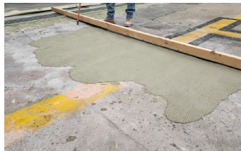
Elephant Armor® is applied in 3 panels to fill and level the repair area.
