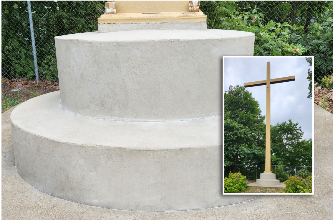
Surface Armor's ease of use and quick set time, allowed the base to be permanently repaired with a minimum disruption to the sanctuary in less than 2 hours!
