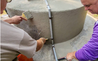
Apply Surface Armor® vertically using a brush, then use a Squeegee Trowel to remove brush marks.
