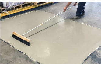
A no-slip broom finish is applied after the second coat of Surface Armor™.
