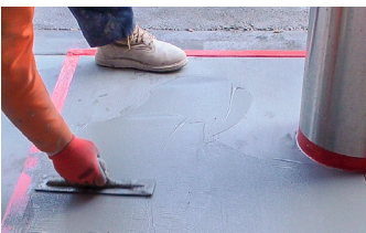
Applying second coat of Surface Armor™ to surface prior to brooming.
