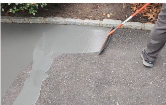
Applying Surface Armor™ is quick and easy with a GST Squeegee Trowel.
