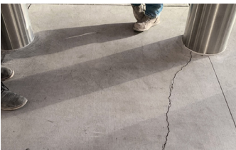
Sidewalk panel prior to crack fill with first Surface Armor™ coat.
