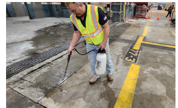
A coat of Ecobeton-USA Vetrofluid® is applied to stabilize the existing concrete.
