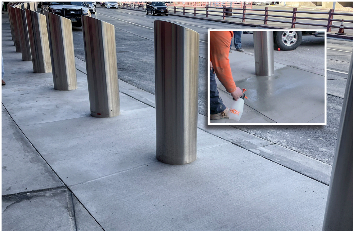
Finished panels showing a new appearance. Inset photo shows Ecobeton-USA Vetrofluid® being applied as the final step of the Surface Armor™ System.
