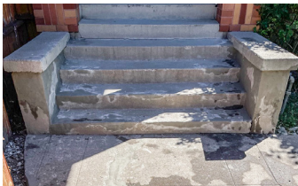
Elephant Armor® reconstruction complete, now ready for Surface Armor™ permanent micro-topping.
