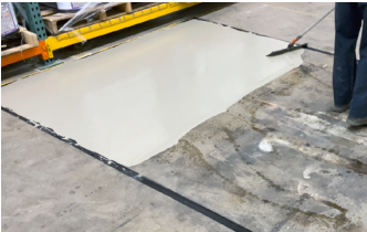
First coat of Surface Armor™ being applied with a GST Squeegee Trowel.
