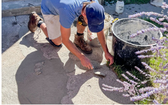
Elephant Armor® DOT used to fill all spalls, deep cracks and displacements. Forming not required.
