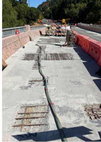
Structural repair area of exposed steel on the bridge deck.
