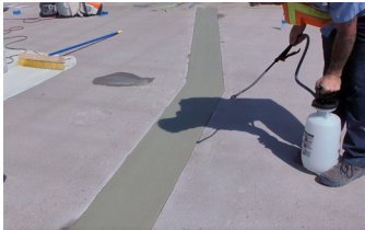
Finishing Elephant Armor® repair with an application of Ecobeton® Vetrofluid®.
