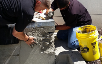
Applying Elephant Armor® to the vertical surface without forming.
