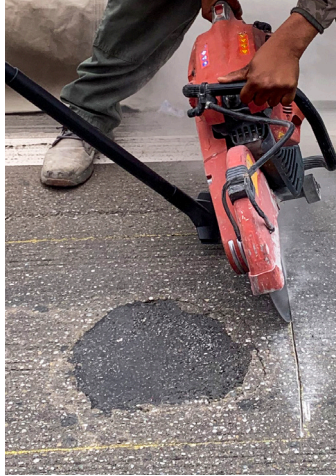
It is important to make clean cuts around the perimeter of area to be repaired.
