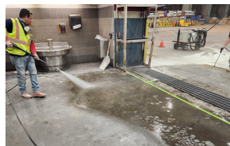
Area to be repaired is washed and all loose material is removed.
