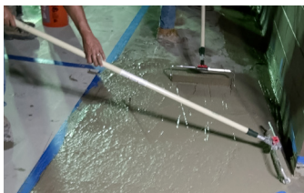
Applying second lift of Elephant Armor®.
