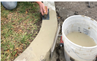
Finishing curb repair with edging tool.
