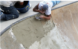
Elephant Armor® applied after primer coat.
