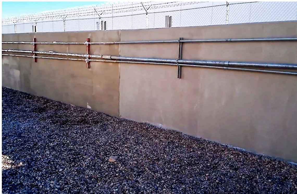
A newly resurfaced CMU block wall with a 'like new' appearance, eliminating the visual cracks and discoloration. The wall is now waterproof and structurally sound.
