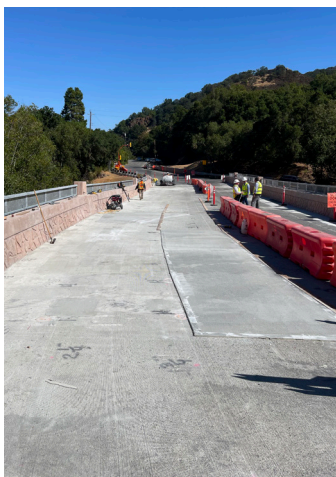
The first overlay is cured and ready for the second 1/2" lift.
