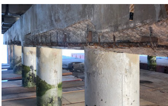
Damaged and unsound concrete removed and prepped for Elephant Armor® placement.
