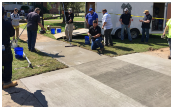
Using a GST Squeegee Trowel prior to applying a broom finish.
