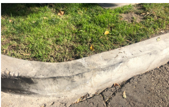
Finished curb can take immediate vehicular abuse.
