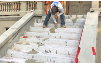
Filling larger cracks prior to full encapsulation.
