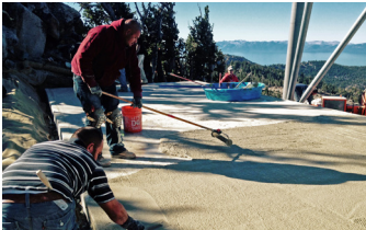
Elephant Armor® applied with GST rollers and trowels.
