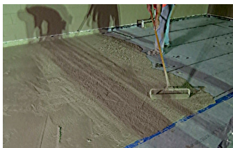
Applying first lift of Elephant Armor® over waterproofing membrane.
