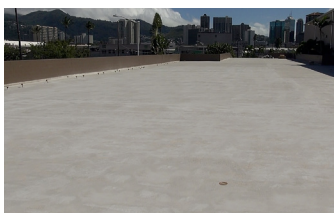
Repair complete and ready for use.
