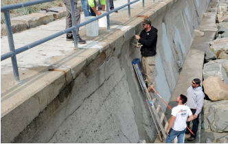
Applying Elephant Armor® to repair area.
