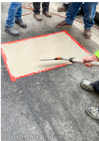
A GST Squeegee Trowel is used to smooth out the Elephant Armor®.
