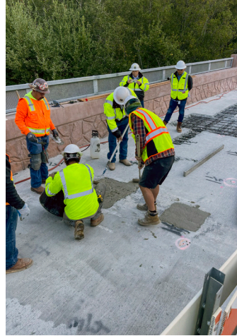
Applying Elephant Armor® as a fill material around the exposed steel.
