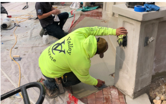
Finishing vertical wall repair.
