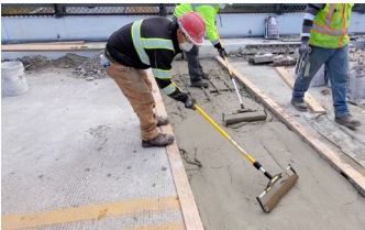
Placement of material using GST Texture Rollers.
