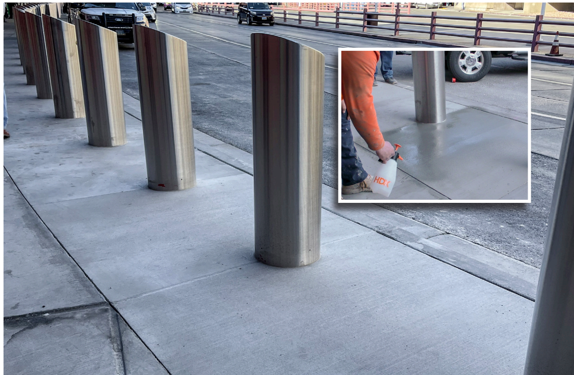
Finished panels showing a new appearance. Inset photo shows Ecobeton-USA Vetrofluid® being applied as the final step of the Surface Armor™ System.
