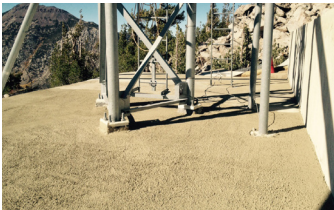
CBS TV Tower completed reconstruction in just 4 days.
