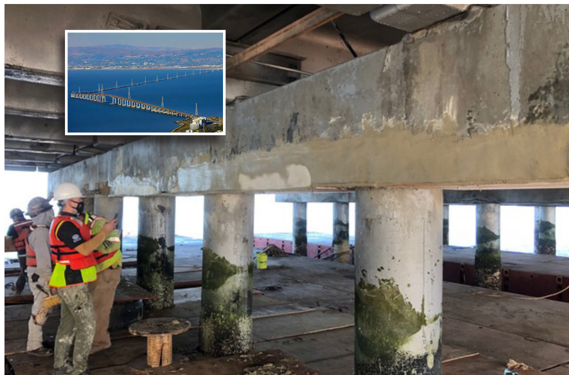
CalTrans using Elephant Armor® DOT on a 3 year project to bring the bridge back to its original specification without having to fully deconstruct and reconstruct the failing 1100 columns.
