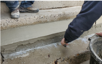
Putting finishing touches on the repair.
