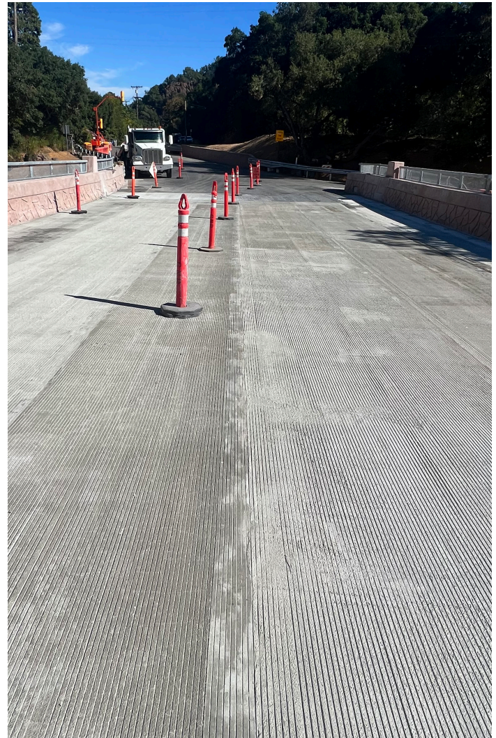
Completed bridge deck resurfacing taking approximately just one week to perform.
