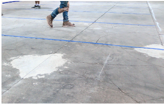
Defining repair area by saw cutting and taping.
