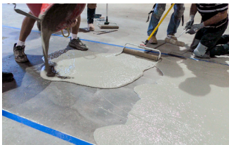
GST Gauged Rollers are used to apply Elephant Armor® at a consistent 1/4" thickness.
