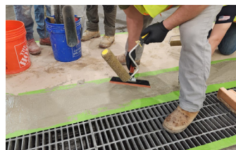
The second damaged area on the outside perimeter of drain is now overlaid with Elephant Armor®.
