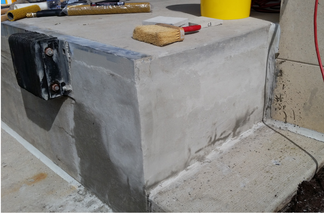
Damaged loading dock repaired without the need of forming and a lengthy interruption of service.
