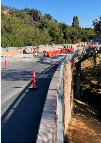
Alimitos Bridge in Santa Clara County, California
