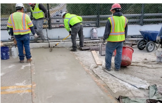
Putting final finish on new bridge link.
