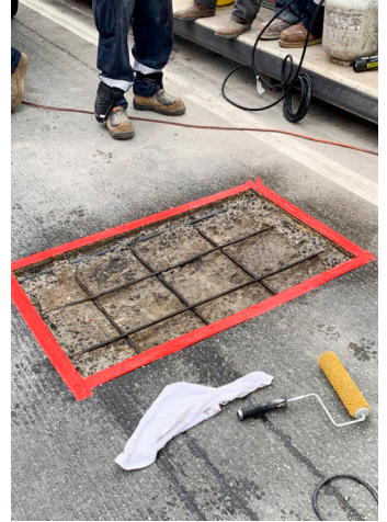
The clean and stable repair area is 'surface saturated dry' (SSD) prior to the placement of Elephant Armor®.
