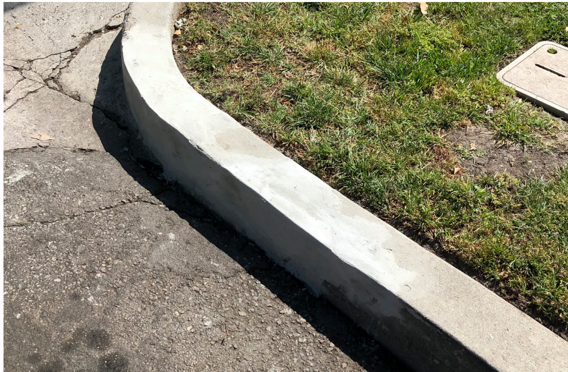
Finished curb repair completed in less than an hour.
