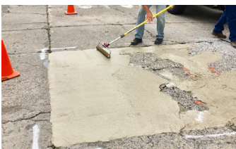
Application of quarter inch Elephant Armor® overlay.
