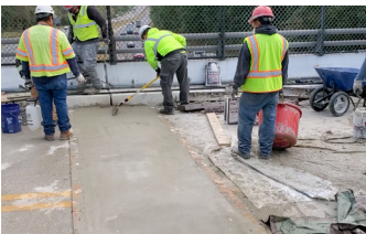
Putting final finish on new bridge link.
