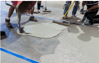
GST Gauged Rollers are used to apply Elephant Armor® at a consistent 1/4" thickness.
