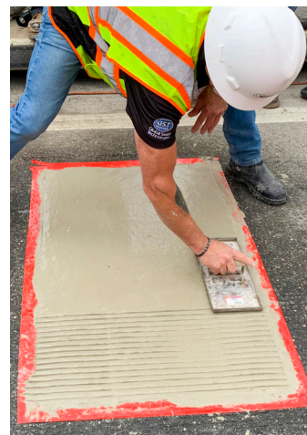
A tining trowel is then applied to the surface to match the existing bridge deck grooved surface.
