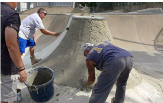
Elephant Armor® applied with GST Rollers and trowels without forming.
