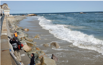
Repair completed during low tide cycle.
