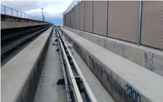
2 coats of Surface Armor™ were applied for durability and texture.
