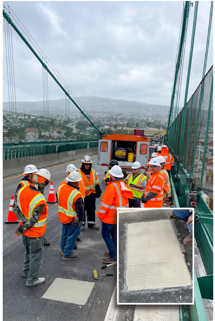
Elephant Armor's ease of use and quick set time, allowed the pothole to be permanently repaired with a minimum disruption to bridge traffic. This lane was back to service in less than 3 hours!
