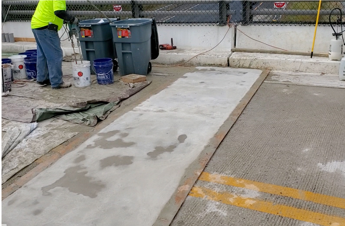
Bridge link construction completed in just 4 hours. Elephant Armor® was chosen due to its high compressive, flexural and tensile strength. Its fast setting properties allow for minimal shut down time and a quick return to service.
