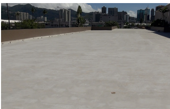
Repair complete and ready for use.
