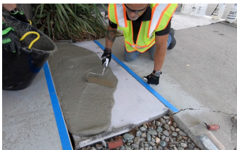
Applying Elephant Armor® using a GST Texture Roller.
