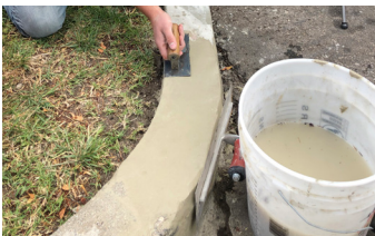
Finishing curb repair with edging tool.
