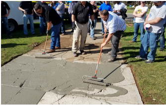
Applying a slurry coat and crack fill with Elephant Armor®.
