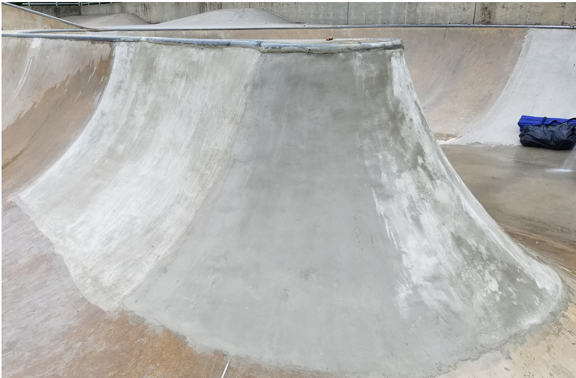
Overlay of degraded failing concrete completed with Elephant Armor®.
