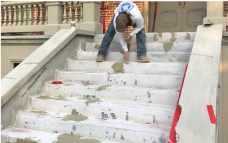
Filling larger cracks prior to full encapsulation.
