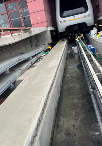
Ecobeton®-USA Vetrofluid® sprayed on prior to Surface Armor™ application.
