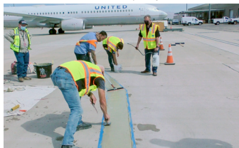
Elephant Armor® cap is placed using an edging trowel and squeegee.
