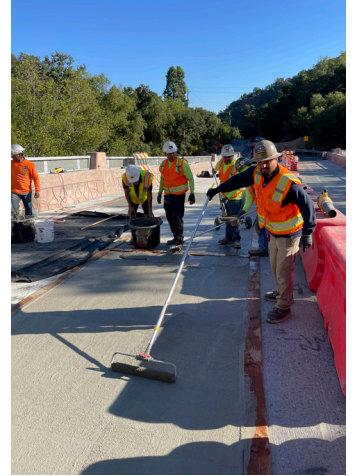
The first 1/2" lift overlay being applied to the bridge deck.
