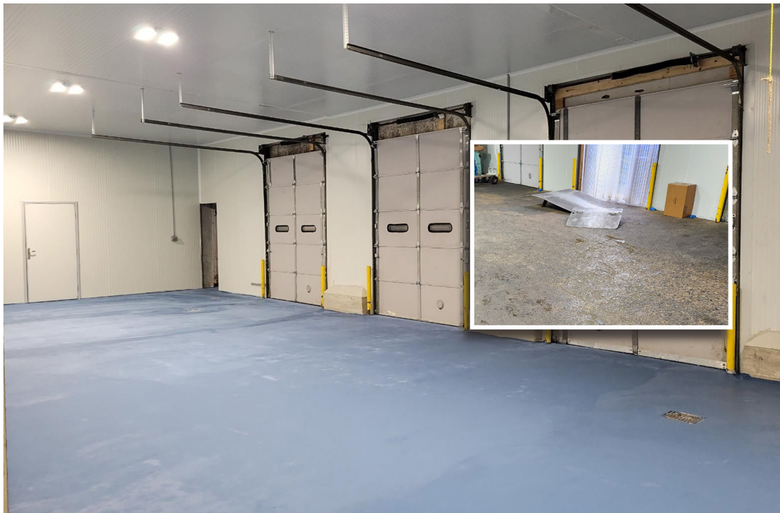
Clean floor with Pro-Grade Cleaner before applying Ecobeton® Vetrofluid.
