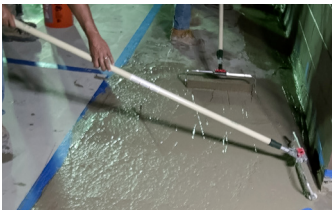
Applying second lift of Elephant Armor®.
