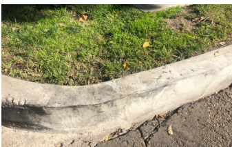
Finished curb can take immediate vehicular abuse.
