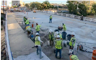
Placing Elephant Armor® using GST specialized tools.
