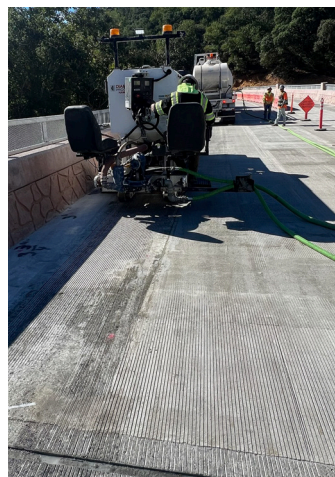
After the second lift has cured, a grooving machine applies the specified texture.
