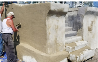
Placing Elephant Armor® on vertical wall.
