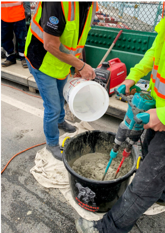
Elephant Armor® is easy to prepare, just add water. A ColloMix Xo 55 Duo is required for generating the high shear needed to achieve a homogenous mix.
