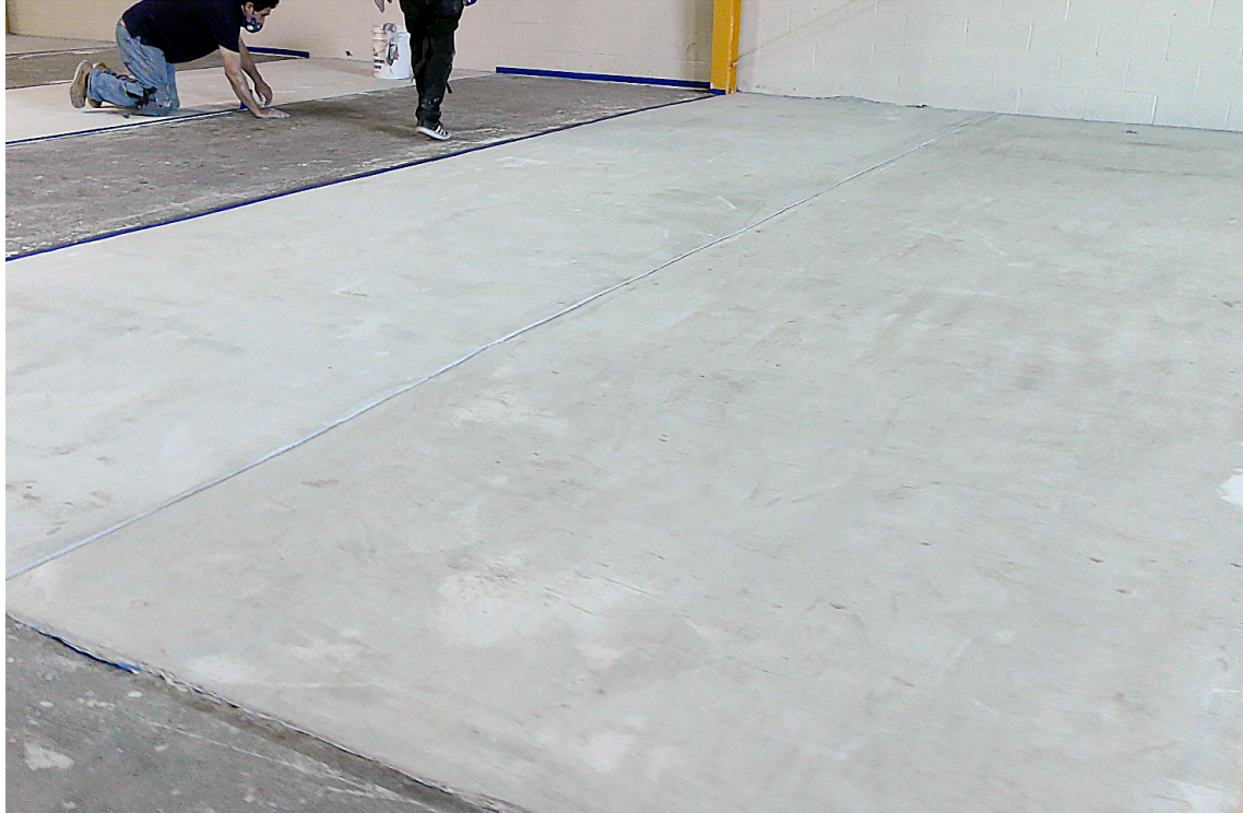
The installation was completed in sections allowing for uninterrupted use of the warehouse, saving 80% of the original remove and replace estimate.
