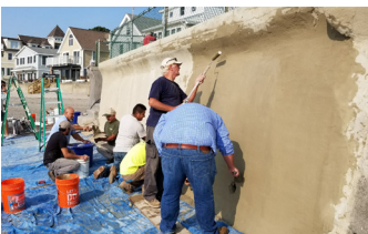
Using GST Texture Roller for final placement.
