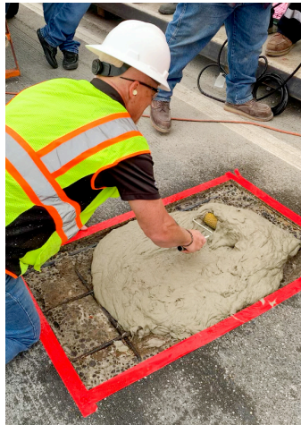
A GST Textured Roller is used to place and evenly spread out the high fiber mix design of Elephant Armor®.
