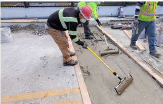
Placement of material using GST Texture Rollers.
