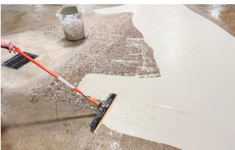
Applying Surface Armor® is quick and easy with a GST Squeegee Trowel.
