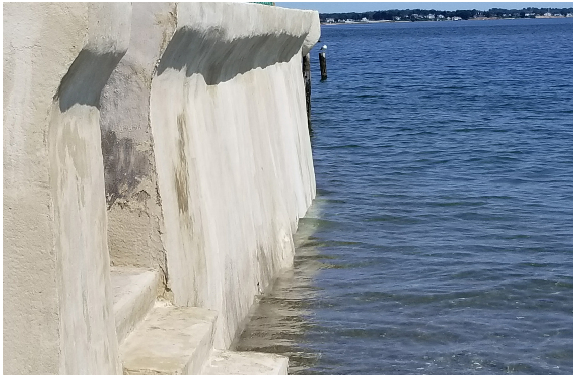
Full degraded seawall encapsulation completed between tides.
