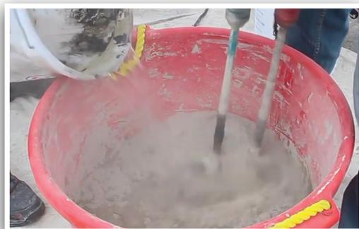
4. Add 90% of the pre-measured water directly over the paddles of the mixer while running.
